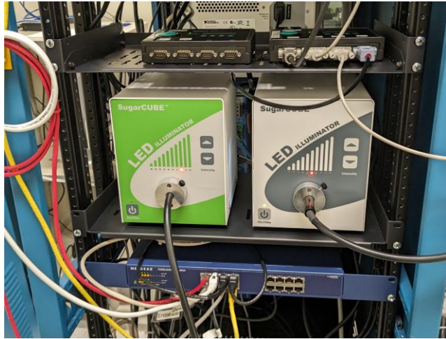
LED illuminators (525 nm and white)
